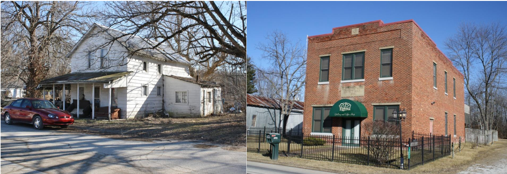
Figures 32-33. Henderson House (c. 1910) and former Bean Blossom Masonic Lodge No. 527 (1922)
