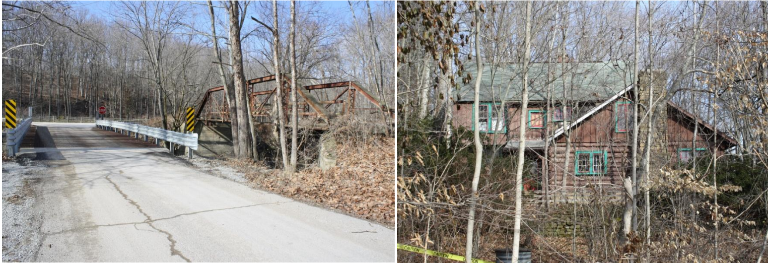
Figures 46-47. Steel truss bridge on Yellowwood Road (c. 1910-20) and Stewart-Cagle House (1937; c. 1950)
