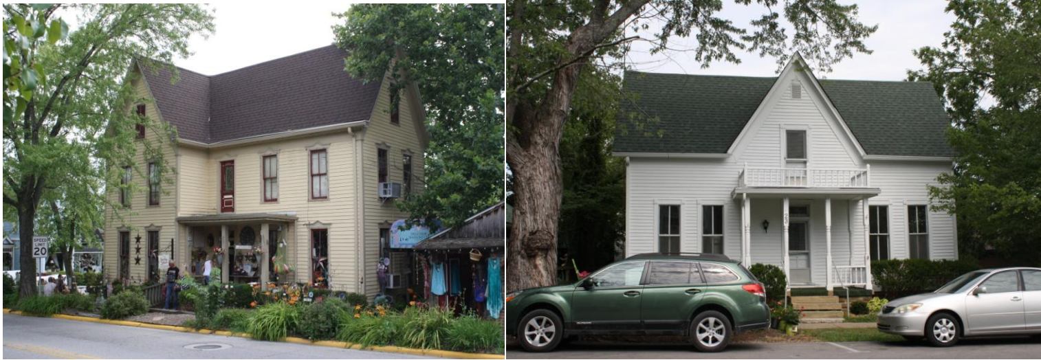
Figures 77-78. Bartley-Gibson-Hohenberger House (c. 1875-80) and Tilton House (c. 1875)
