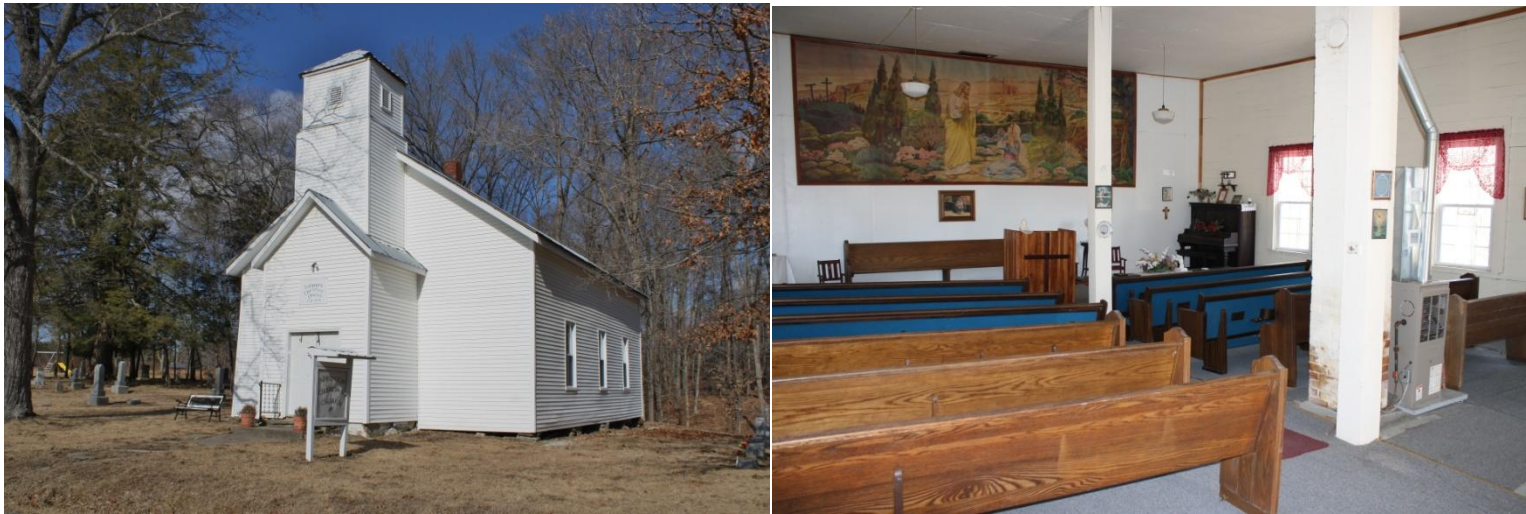
Figures 22-23. Sprunica Christian Church—rehabilitated exterior and interior (c. 1870)
